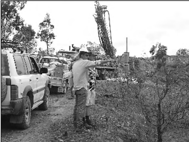
Drilling in progress
